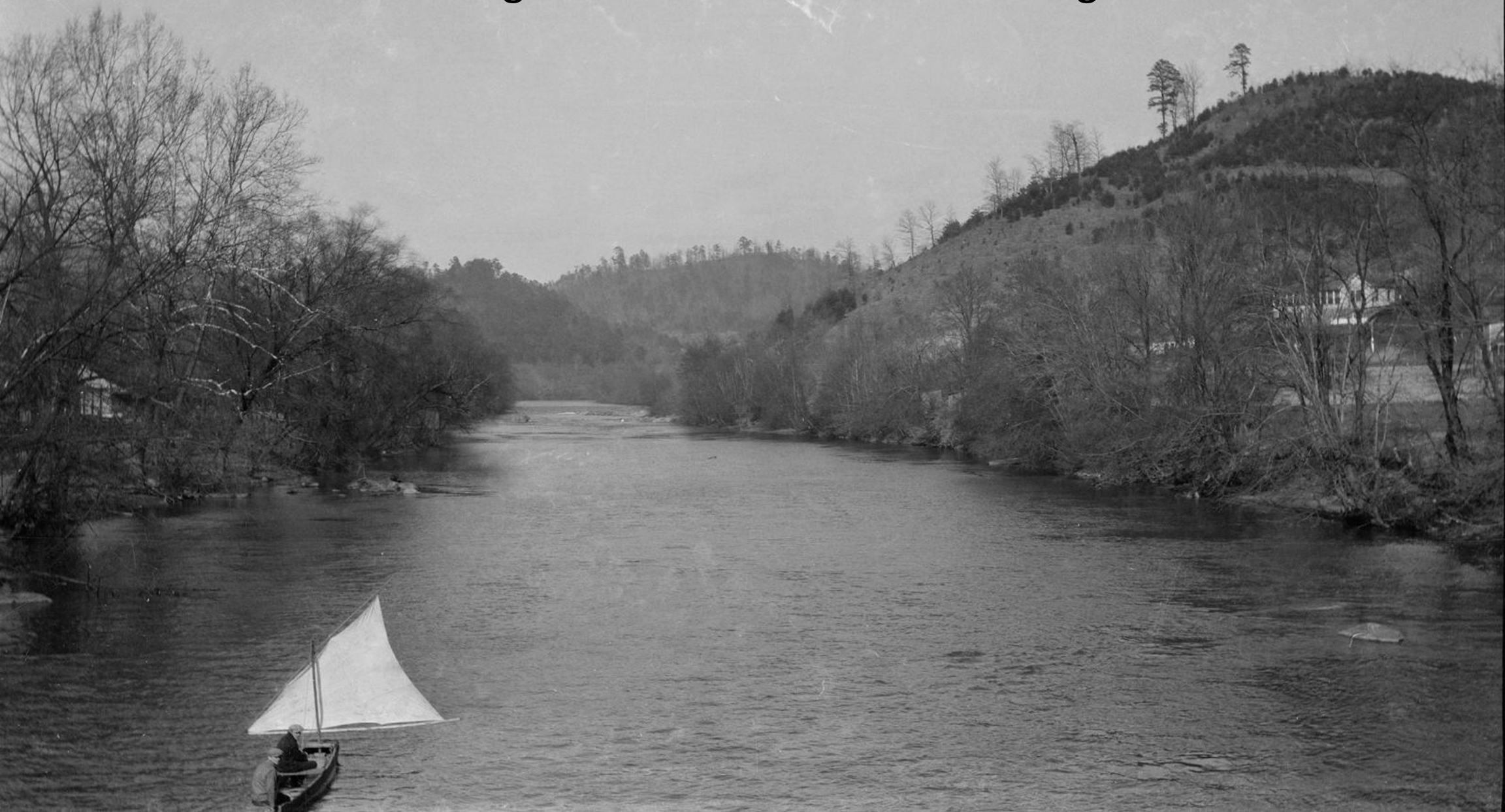
Looking east from Everett Street bridge
