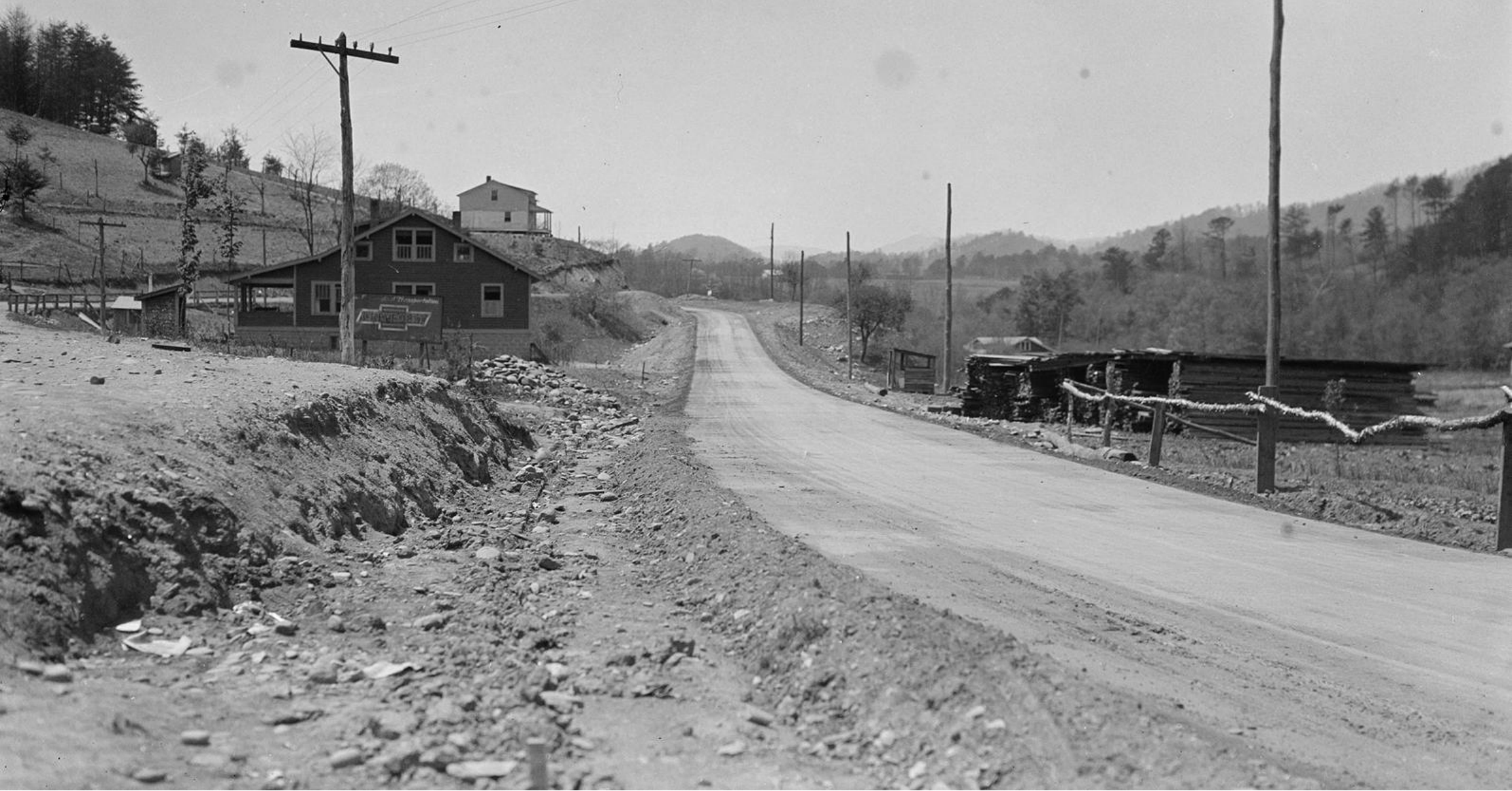
View to the west along NC 10 from near current Hot Spot
